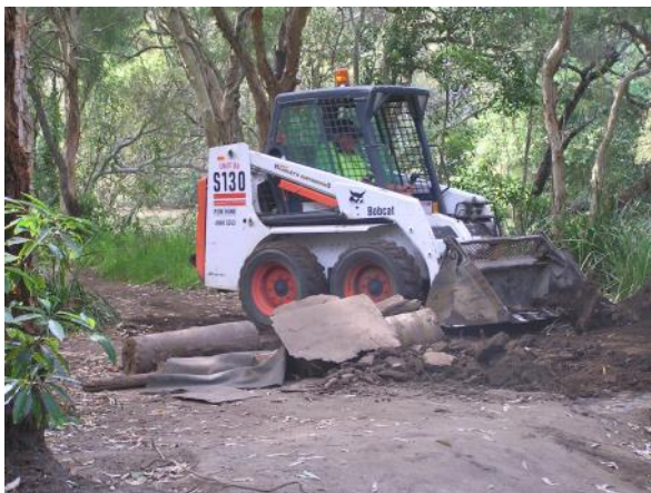
Earthmoving equipment was used to reshape the disturbed surface.
