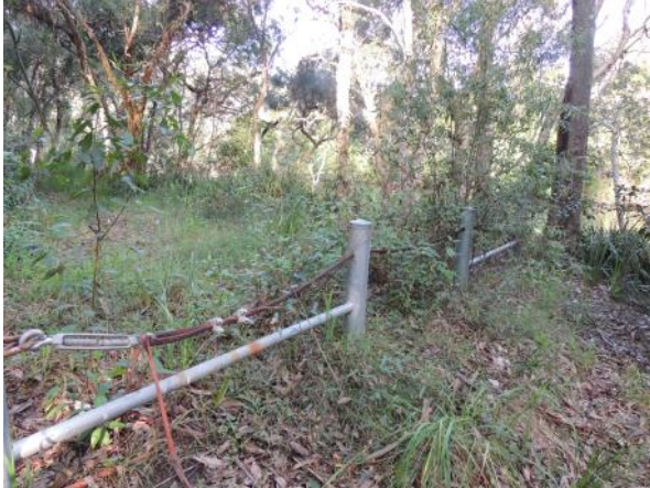
Steel posts and cables were placed at intervals to discourage bike riders.
