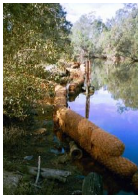
Ecologs placed along South Creek to protect the bank from erosion, 2000
