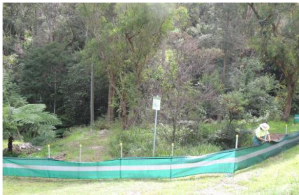
Placing protective fencing on Bucklee site on Warner's Creek, 2014
