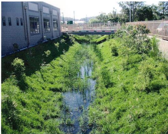
North Creek looking upstream towards King Street: Landcare has been unable to plant on this site because it is inaccessible. The growth of weeds and other plants in the channel has, nevertheless, helped filter nutrients and sediment from the runoff water and provide habitat.
