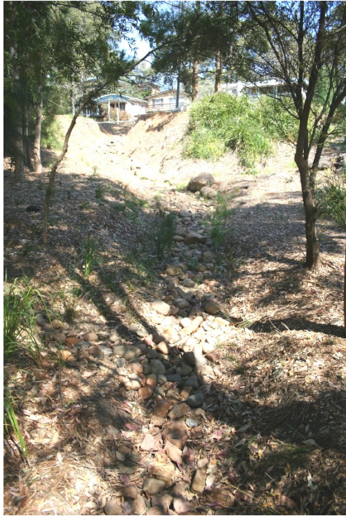
October 2009, Creek line after restoration work completed.
